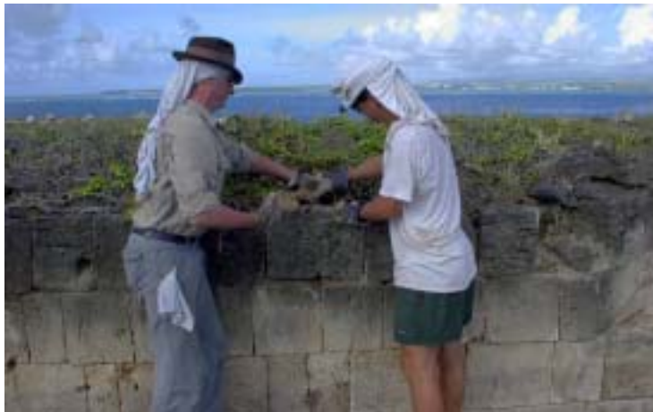
Conservation First Aid... Bradley and Jonathan pushing back into position the displaced stone seen at center left in the previous photo. (03jv1304)
