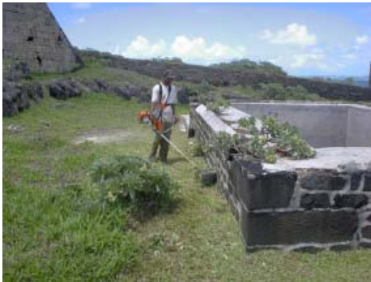
Figure 14. A grass-cutter with nylon line is ideal for cutting back creeping vegetation. (04jv0205)
