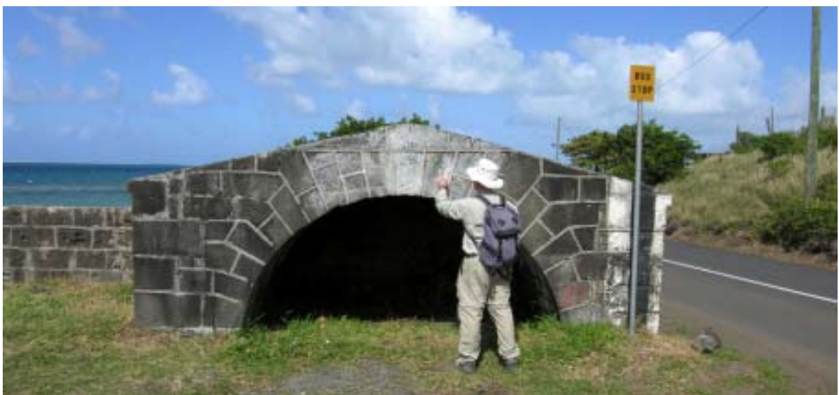
Figure 33. The vault at the southern end of the battery was documented with the help of digital photos and control points for photo-rectification. (md05nc0101)
