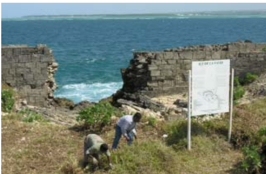
Figure 8. Workmen were employed to clean up the islet, clear vegetation and help with heavy excavation work and backfilling. (mp05nc1209)
