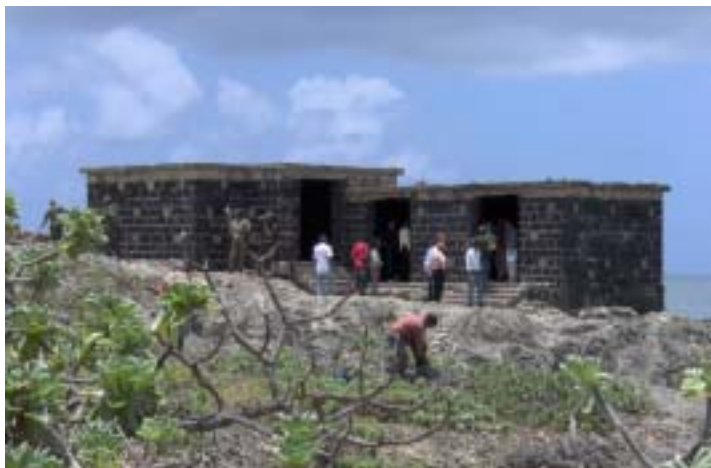
Figure 34. The Searchlight Building was altered and reused during WW II. (mp06nc0881)
