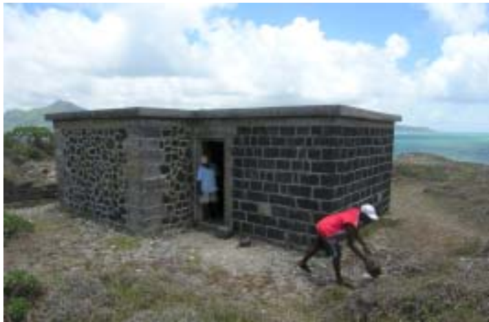
Figure 33. The Central building clearly built in two phases. (mp06nc0505)
